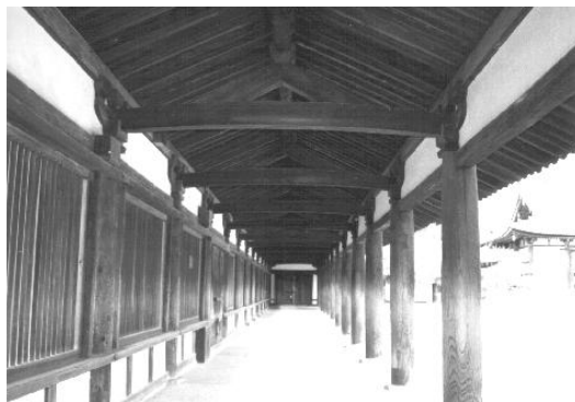
Figure 2: Curved beams as an original shape of KOURYOU
