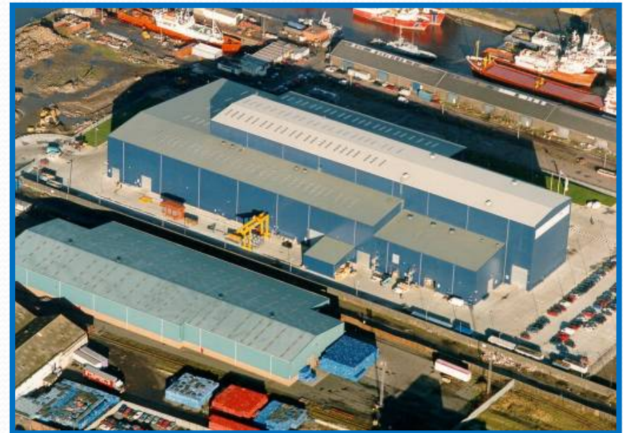
Leith-Edinburgh-Scotland – PWP plant and offices
