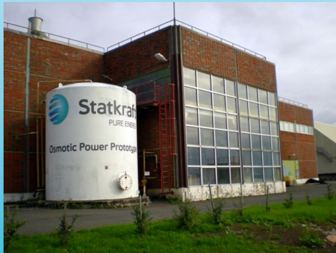
Statkraft's Osmotic Power Prototype, Oslo Operational since October 2009
